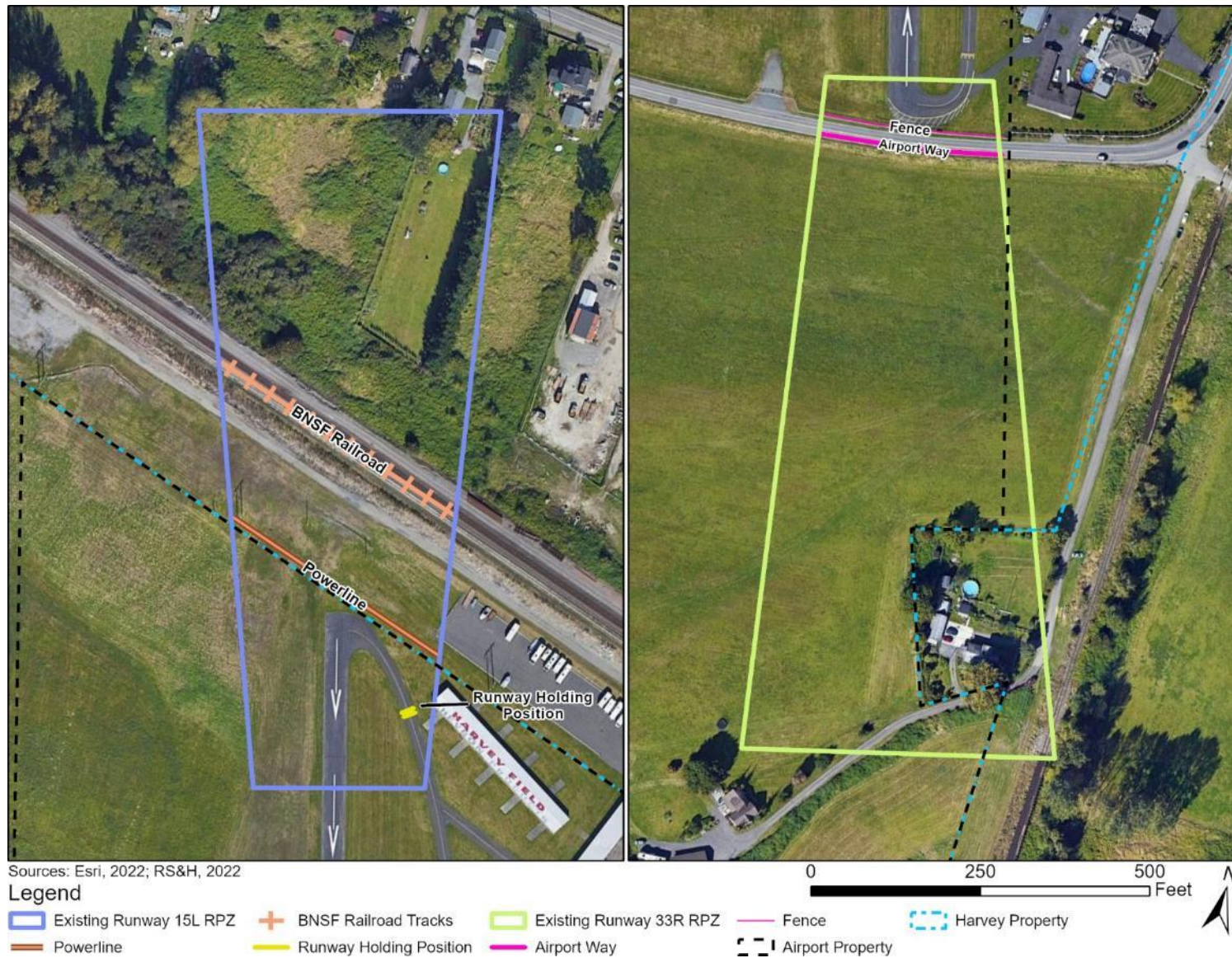
Figure 1-6 Existing Non-standard Runway 15L/33R Runway Protection Zone Obstructions
